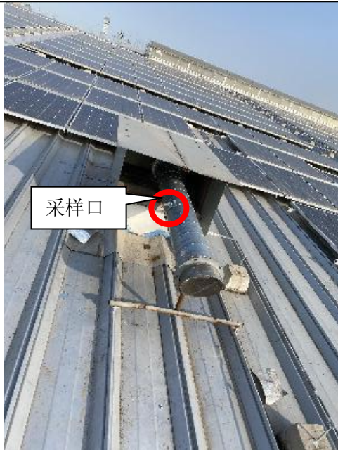
总装废气排气筒 DA006 15m
