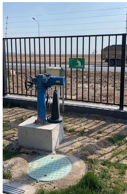
罐区废液收集切换阀
